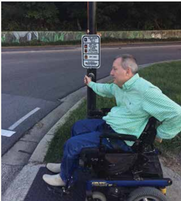
Using newly installed crosswalk
